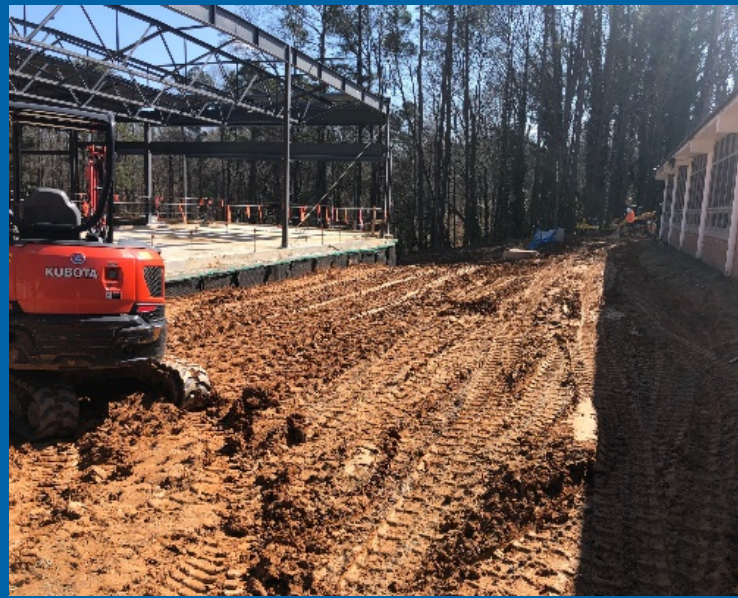
South Gymnasium Wall Backfill
