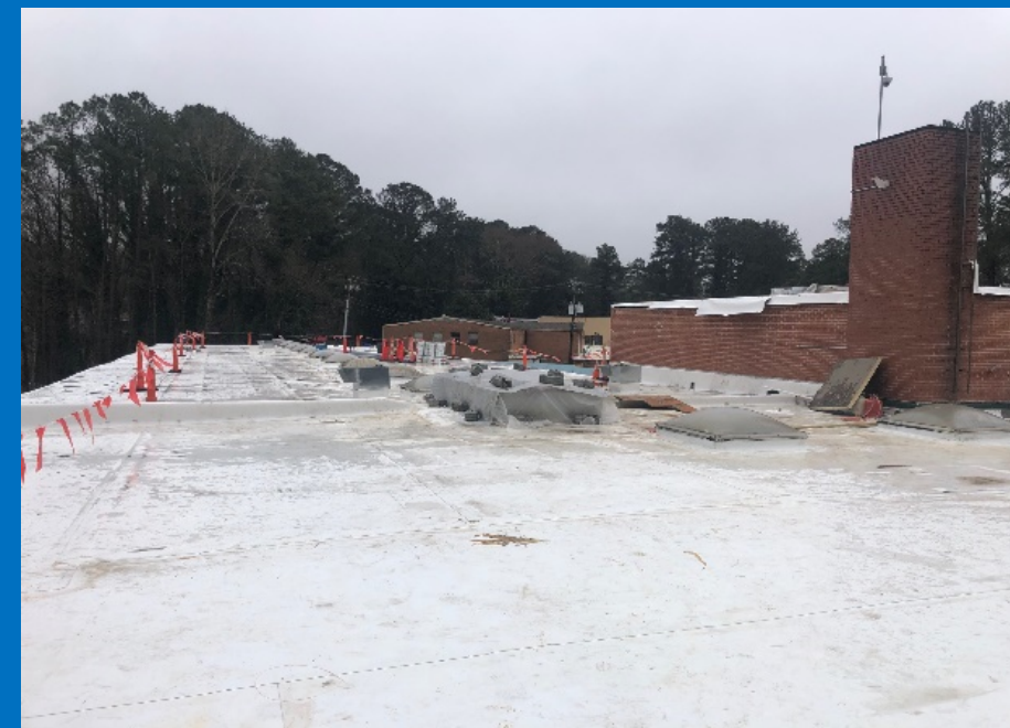
TPO Roofing Replacement
